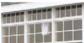
Transom Windows (above windows)
