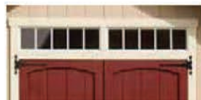
Transom Windows (above doors)
